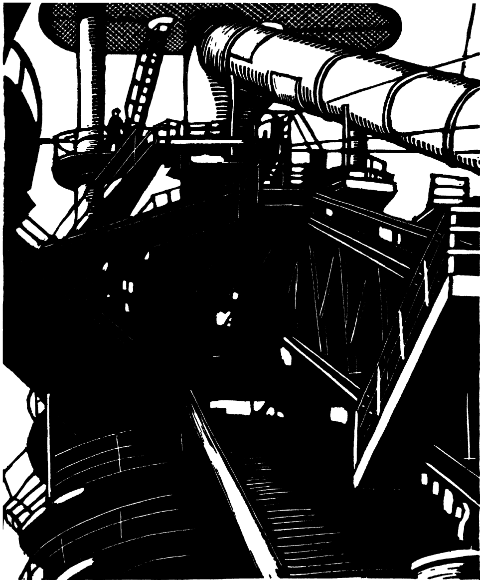
BLAST FURNACE NO. 4 OF THE MAKEIEV FACTORY. THIS IS THE LARGEST BLAST FURNACE IN THE UNION AT PRESENT. LIQUID PIG-IRON IS Poured INTO THE TUB WHICH STANDS ON THE PLATFORM. THE TUB THEN GOES UP, TURNS OVER, AND POURS THE ORE STRAIGHT INTO THE MOUTH OF THE GIANT BLAST FURNACE
